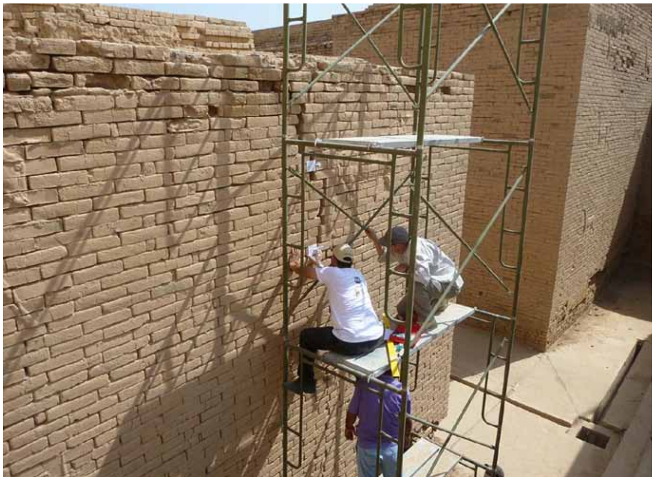
Emergency shoring being erected at Nabu-sha-Khare Temple
