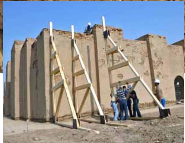
Crack monitors were installed at the Ishtar Gate, left, to record shifting of the fragile ruins. A WMF conservator, above, documents decomposing brick at the base of the temple walls. Emergency shoring, right, was installed at Nabu-sha-Khare Temple. Laser scanning allowed the creation of detailed digital models, below, used in documentation and planning.
