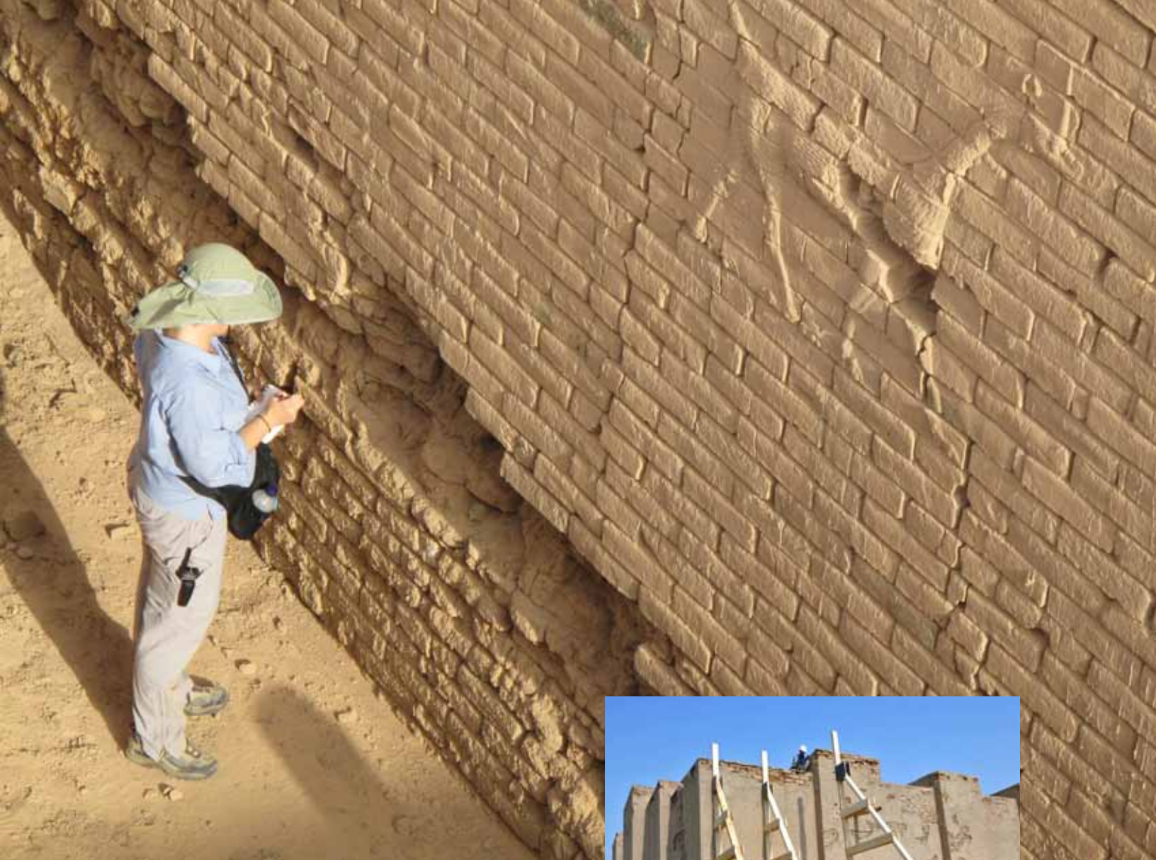
Crack monitors were installed at the Ishtar Gate, left, to record shifting of the fragile ruins. A WMF conservator, above, documents decomposing brick at the base of the temple walls. Emergency shoring, right, was installed at Nabu-sha-Khare Temple. Laser scanning allowed the creation of detailed digital models, below, used in documentation and planning.
